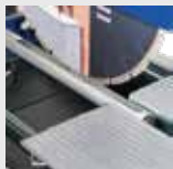
dust extraction at the saw cut
