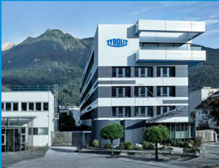
TYROLIT headquarters in Schwaz (Austria)
